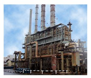
The **Catalytic Reforming Unit** processes the heavy naphtha stream to make it more suitable for the production of motor gasoline. The nominal design charge capacity of this unit is 30,000 **BPD** of heavy naphtha.
