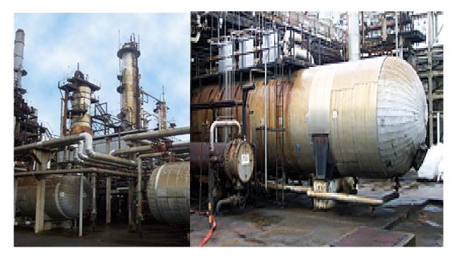
The function of the Crude Distillation Unit is to provide primary separation of the crude oil and natural gasoline feed-stocks for subsequent processing by downstream units. The charge capacity of this unit is 142,000 **Barrels per day (BPD)** of crude oil and 10,000 **BPD** of natural gasoline.
