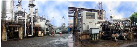
The Hydrocracker Unit processes gas oil, primarily from the **Crude Distillation Unit** and the **Delayed Coking Unit**, to convert it into gasoline, jet, and diesel blendstocks. The nominal design charge capacity of this unit is 40,000 **BPD** of gas oil.
