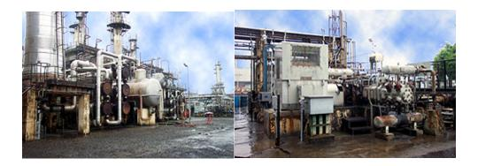
The **Distillate Hydrotreater Unit** reduces the levels of sulfur and other contaminants in kerosene and diesel fuel products to meet regulatory specifications. The nominal design charge capacity of this unit is 34,000 **BPD** of distillate feedstock. The unit will be capable of reducing the sulfur content in the liquid fuel products to less than 0.05 percent by weight.
