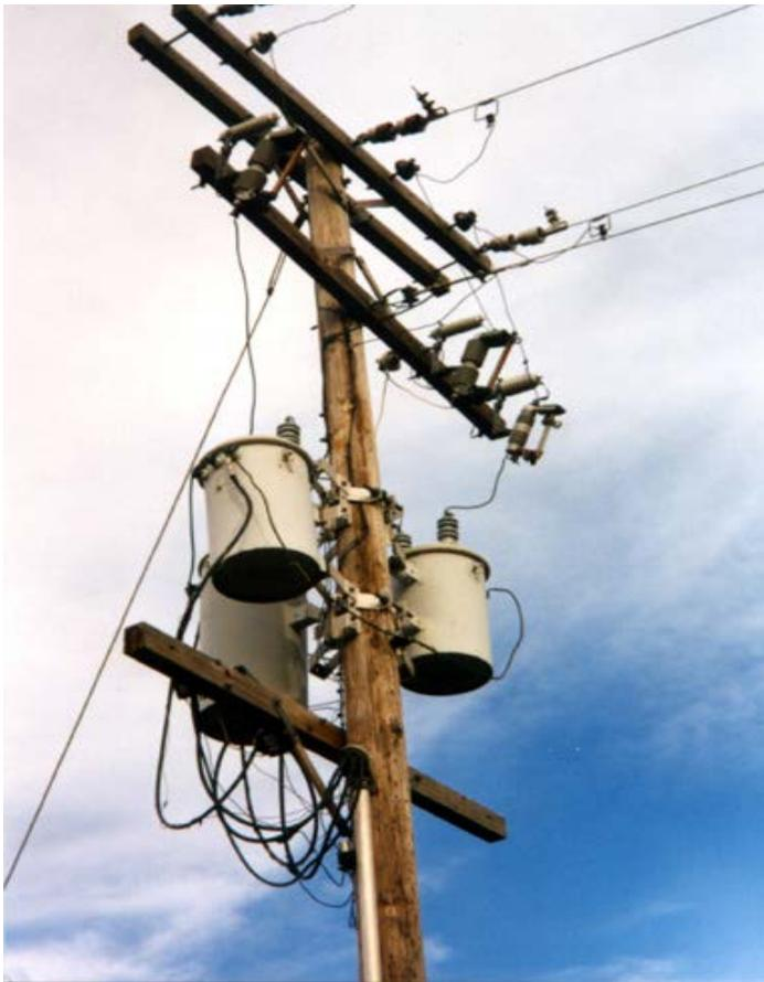
smaller transformers on power line poles reduce the voltage further to the 240V delivered to individual homes
