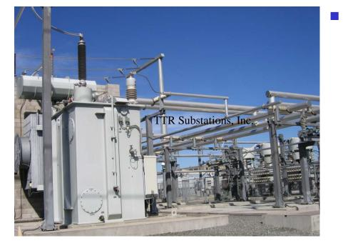
to reduce the very high voltages from the transmission lines (>100kV) to intermediate voltages used to serve an individual town or section of a city (typically 66 kV or 33 kV)
