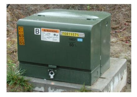
smaller transformers: pedestal mounted, green boxes on the ground) reduce the voltage further to the 240V delivered to individual homes
